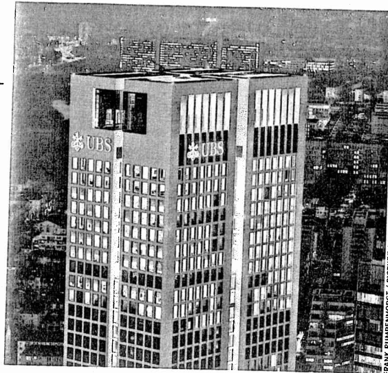
UBS-Tower in Frankfurt am Main
